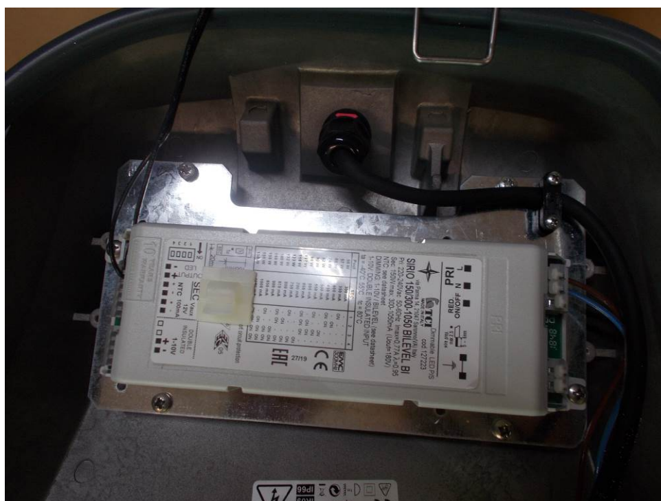
Pic.9: internal view
